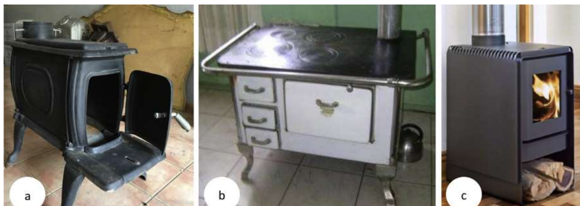
Fig. 4. Most common wood-stoves used in Valdivia. Note: (a) “salamandra” wood-stove, (b) wood-burning cooking stove, and (c) slow-burning wood-stove. Source: own elaboration.
